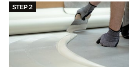
Apply the adhesive to the subfloor in accordance with the adhesive manufacturer's instructions.
