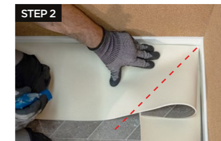
Place the hook blade point in the corner and cut until outside.
