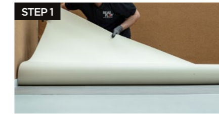
Turn back the first piece of flooring to expose about half of the subfloor.
