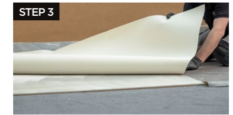
Allow the recommended drying time and then reposition the flooring material over the prepared subfloor.
